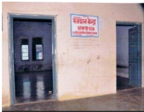
Building Front View
