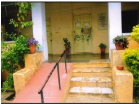
Building Front View
