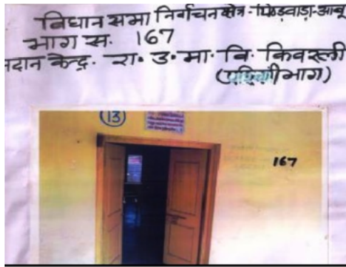
Building Front View
