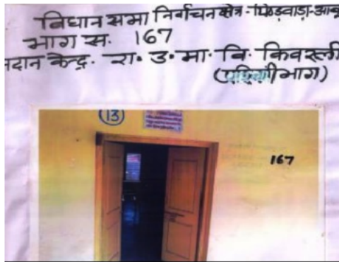
Building Front View
