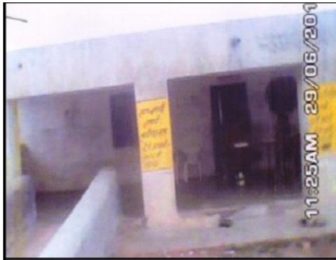
Building Front View
