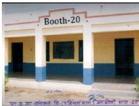
Building Front View
