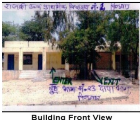
Building Front View
