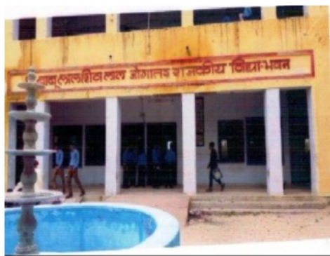
Building Front View
