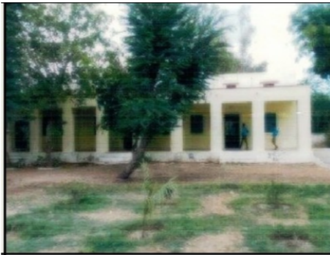
Building Front View
