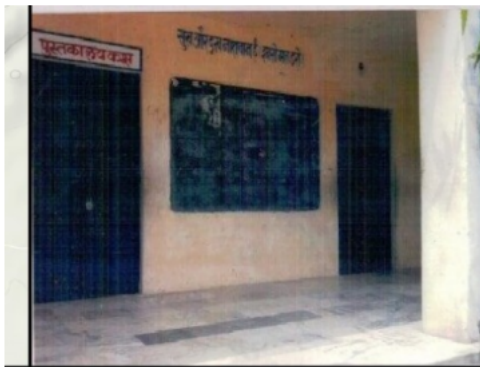
Building Front View
