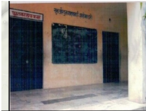
Building Front View
