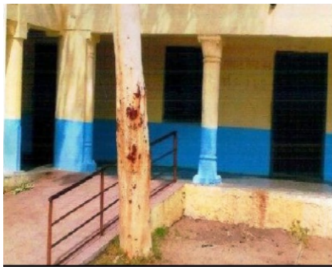
Building Front View
