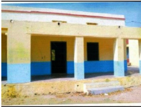
Building Front View
