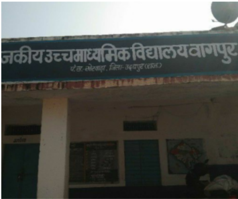
Polling Station Front View
