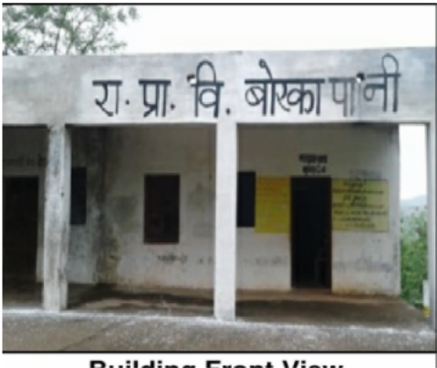
Building Front View
