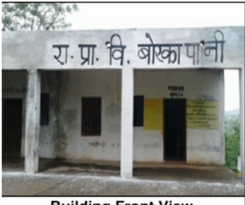
Building Front View
