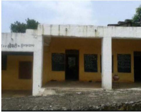
Building Front View
