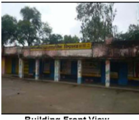
Building Front View
