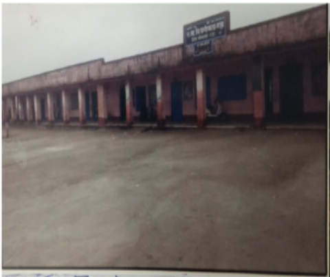
Polling Station Building Front View
