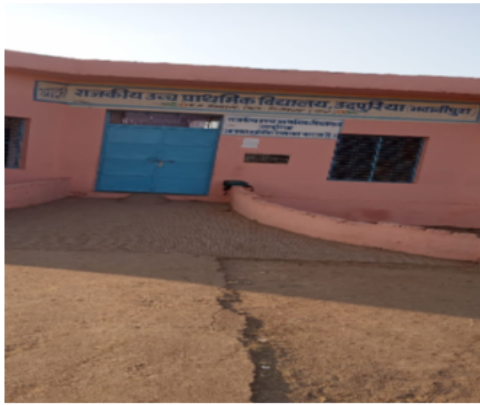
Polling Station Building Front View
