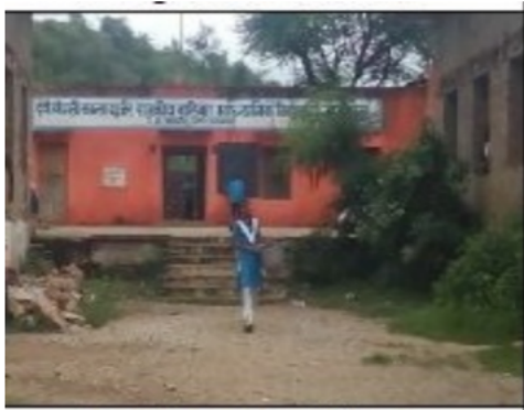
Building Front View
