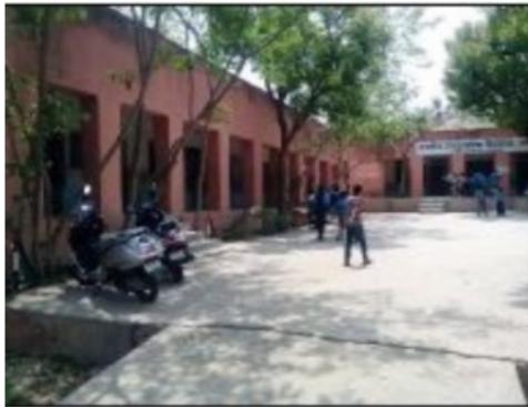
Building Front View
