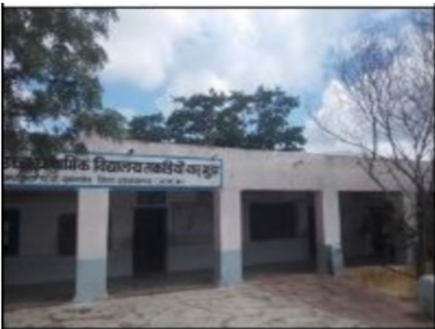
Building Front View
