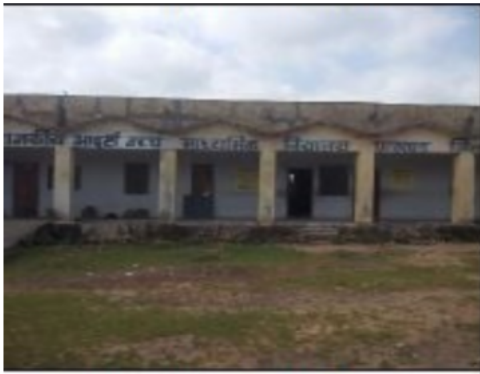
Building Front View
