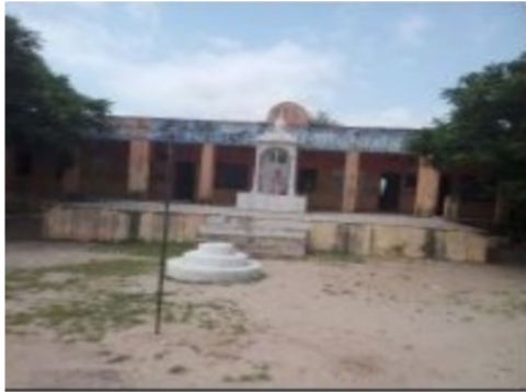
Building Front View
