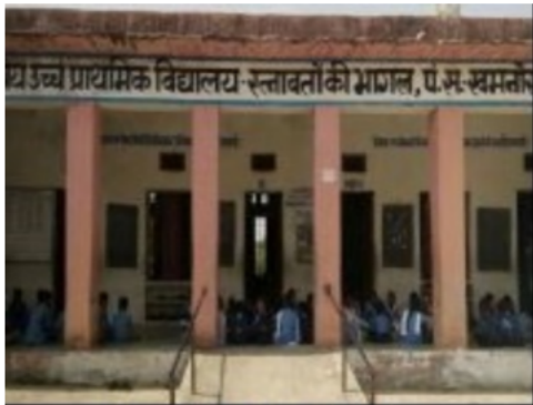
Building Front View
