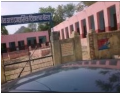
Building Front View
