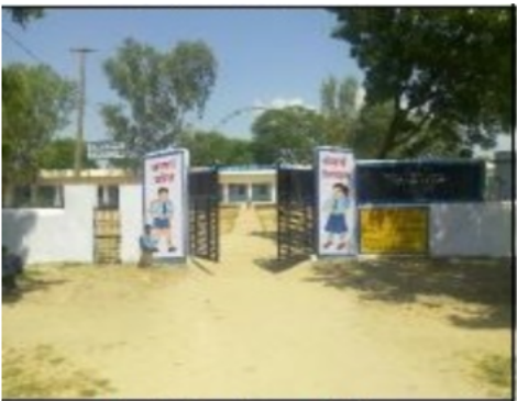
Building Front View
