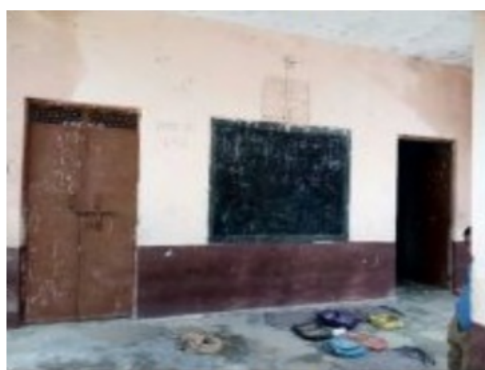
Building Front View
