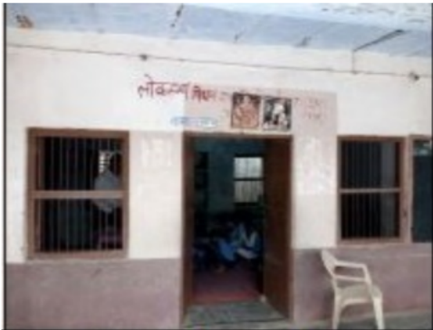
Building Front View
