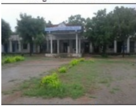
Building Front View
