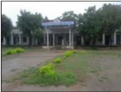
Building Front View
