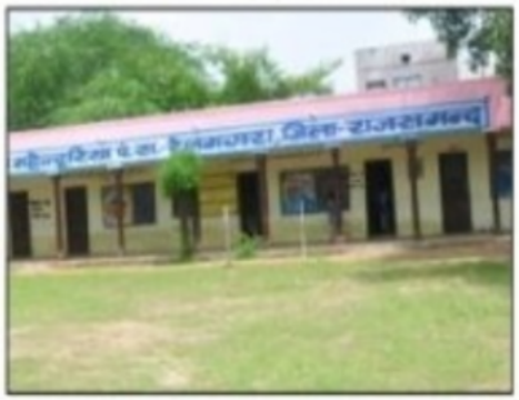
Building Front View
