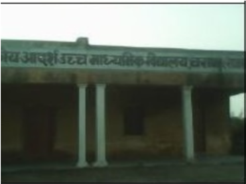
Building Front View
