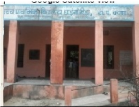
Building Front View
