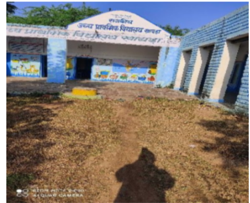
Polling Station Front View
