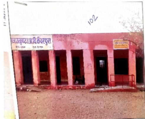
Polling Station Front View
