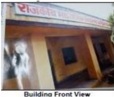
Building Front View
