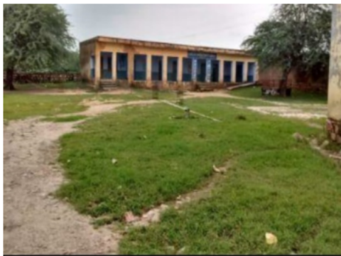
Building Front View
