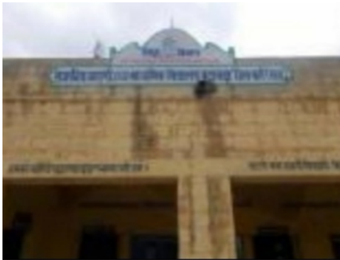
Building Front View
