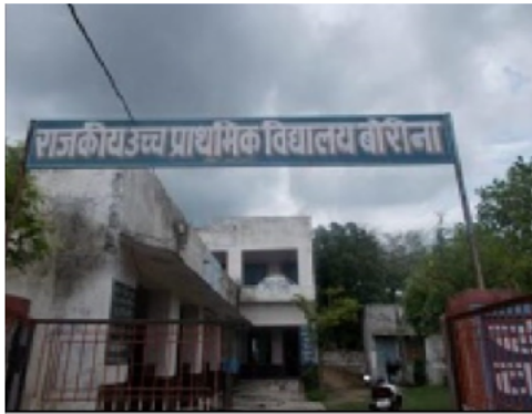
Building Front View
