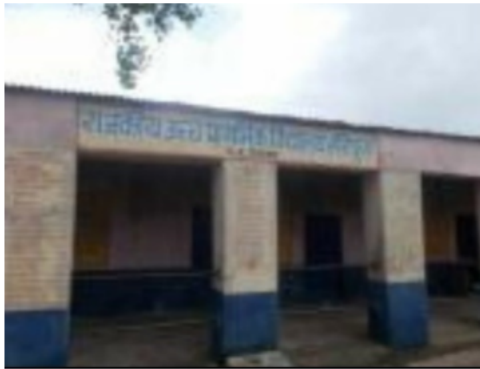
Building Front View
