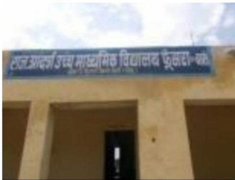
Building Front View
