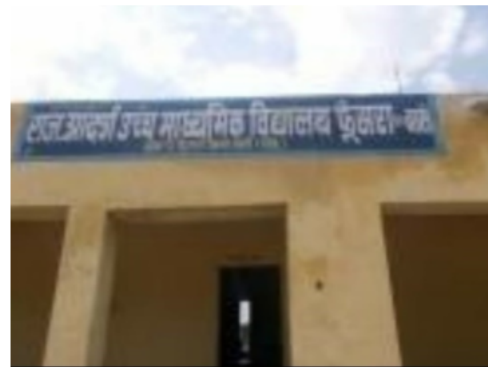
Building Front View
