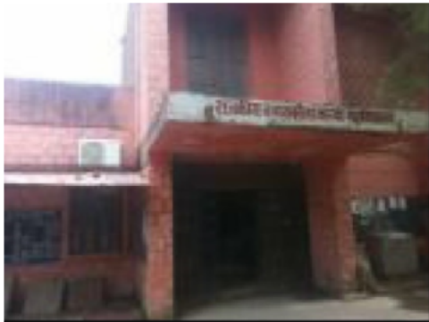
Building Front View
