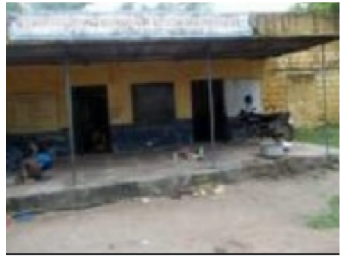
Building Front View
