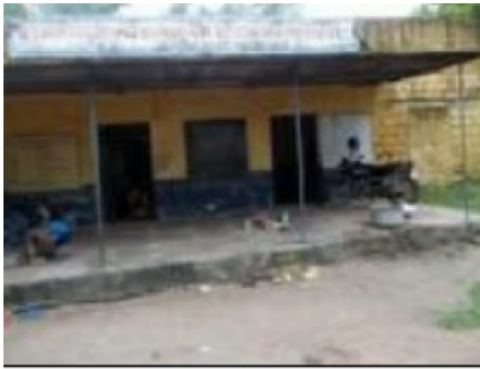
Building Front View
