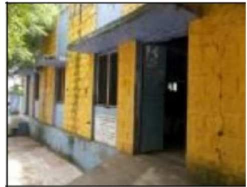
Building Front View
