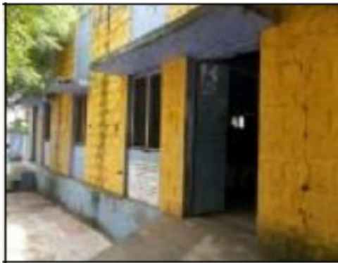
Building Front View
