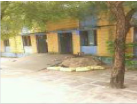
Building Front View
