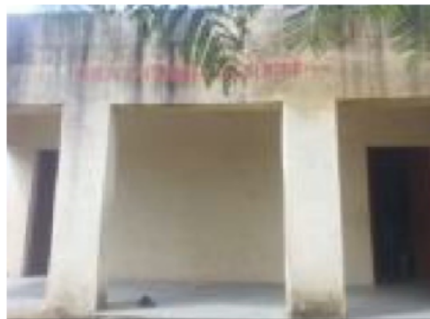
Building Front View
