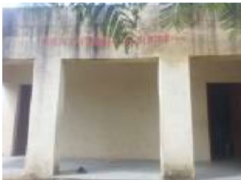
Building Front View
