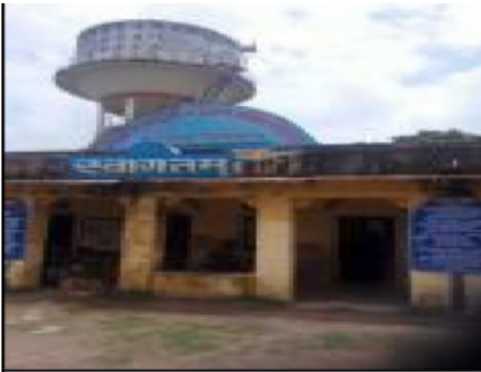
Building Front View
