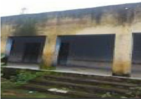
Building Front View
