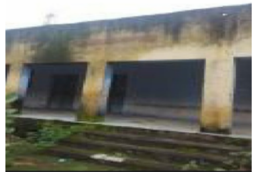
Building Front View
