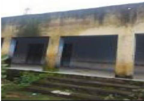
Building Front View
